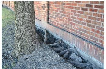
Figure 6. Tree roots growing under foundations (CNT Foundations, 2020)
