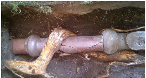
Figure 4. Effects of tree roots on sewer line (911HVAC, 2019)
